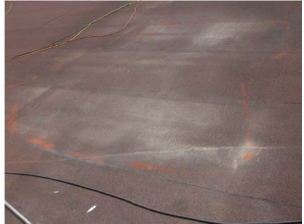
Figure 2. Thermogram and photo pair showing moisture embedded insulation on a single ply flat roof.
